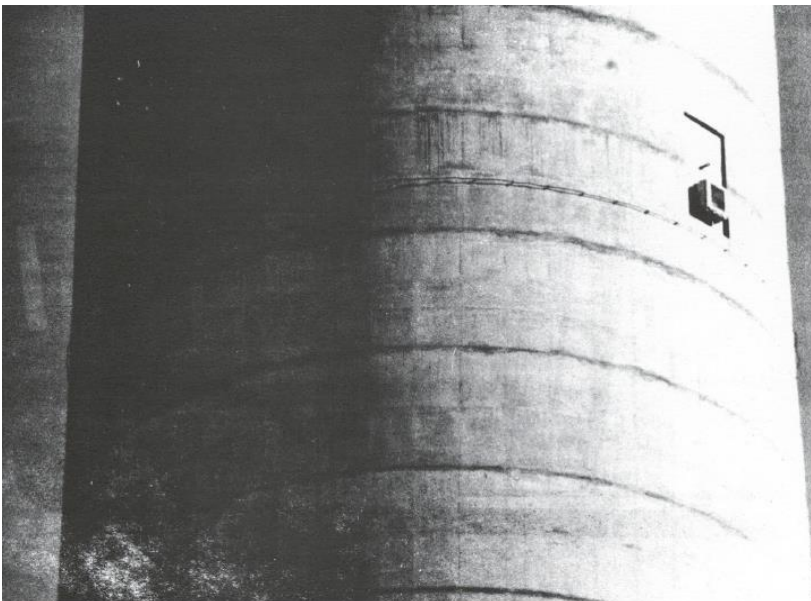
Figure 14-2. High-intensity obstacle lights installed on a chimney
