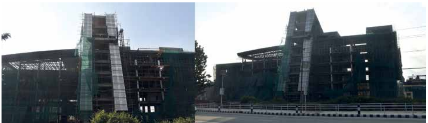
New CAAN Underconstruction Building
